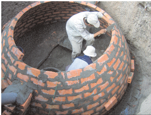
Picture 1: Building a biogas digester in Vietnam Picture 2: Diagram of biogas plant. Source: Journal in Renewable Energy World, “Asia Hits the Gas”.
