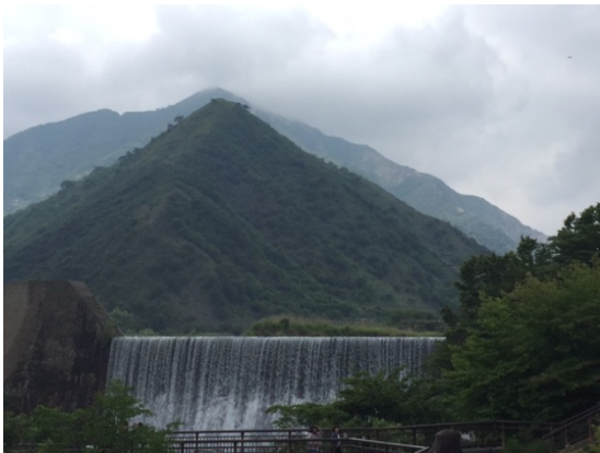
Figure 01: Dam site with the view of mountain range
