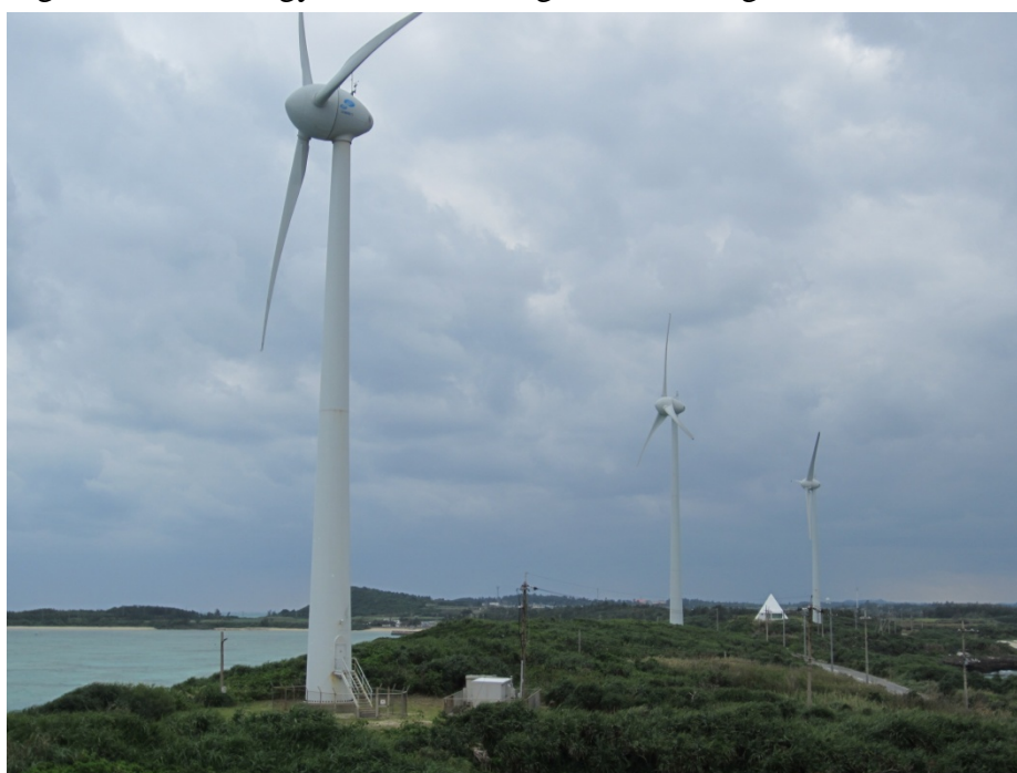
Figure 6: Wind-powered turbine, Karimata Wind Power Demonstration Facility
