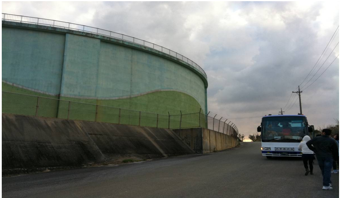
Tank of the water sealing dam, 2011.12.25
