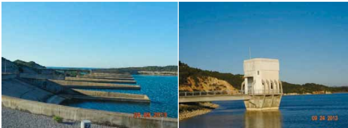
Fig: 2.3.11 The Sidi Al Barak Dam and Reservoir
