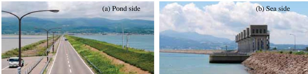
Fig. 2.2 (a) The 7km long Dike separating dam water from seawater, (b) North water gate
