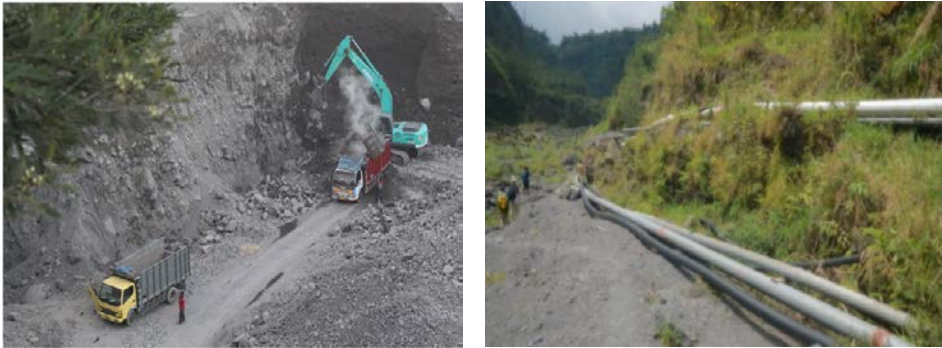
Fig 2 Sand mining and water transportation in Mt. Merapi area
