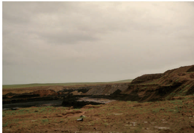
Fig.2.3.2 Removed top soil and coal
