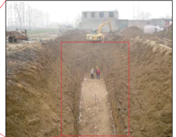
Groove excavation of permeable reactive barrier
